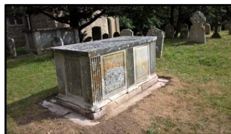
The same view post-restoration, with all parts now safely carrying the load of the heavy recumbent memorial stone.
