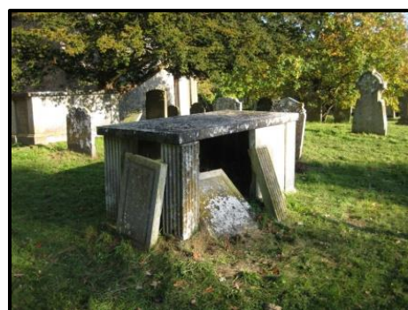
Freeman Denny's tomb before restoration, with collapsed wall panels and displacement of its pillars.
